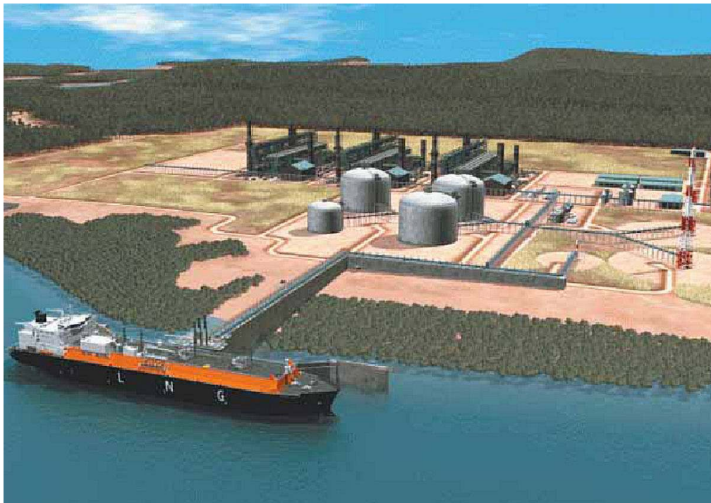
A CSG to LNG conversion plant being built in Gladstone
