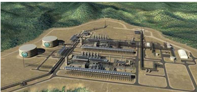
LNG processing plant in Gladstone
